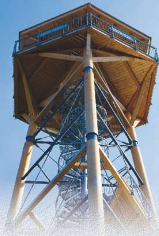
The lookout tower has uniquely just three pillars
